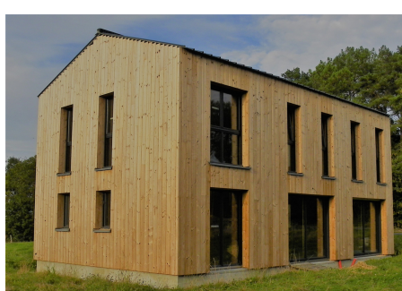
A la pose
