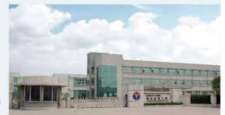
China Jiangsu : Changshu Plant Land Area : 46,620m 2 (501,814ft 2 )
