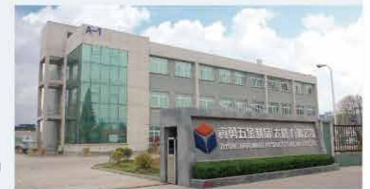
China Jiangsu : Taicang Plant Land Area : 49,253m 2 (530,155ft 2 )
